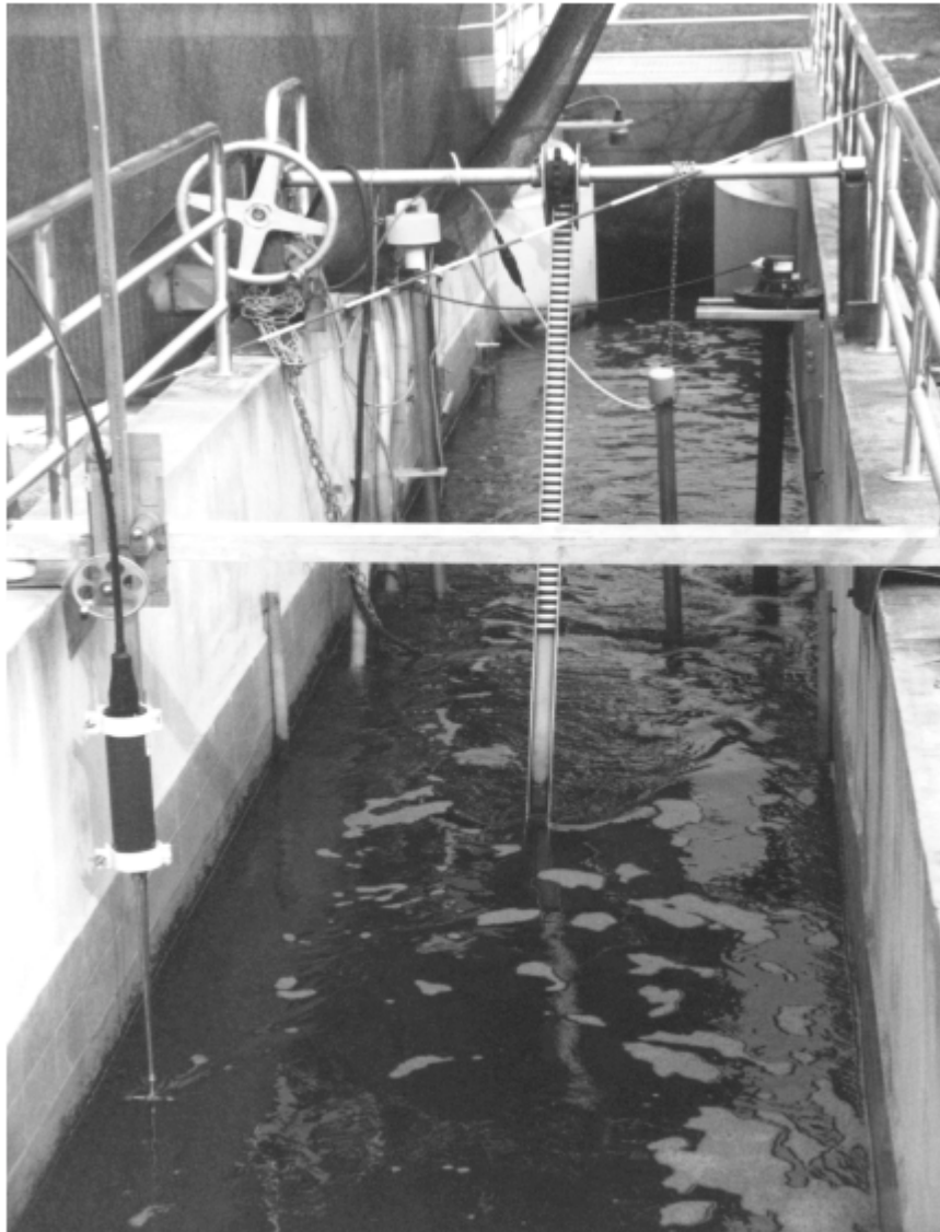
Slika 1. Khafagi Venturi korito na iztoku CČN Domžale. Figure 1. Khafagi Venturi flume on the Domžale WWTP outflow.
